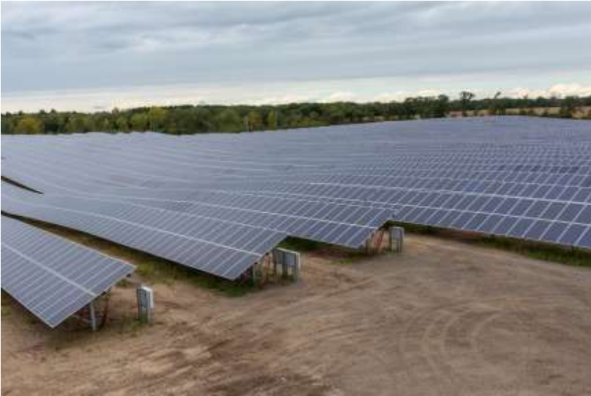
Connexus Energy 6.6 MW Community Solar Garden Athens Township, MN
